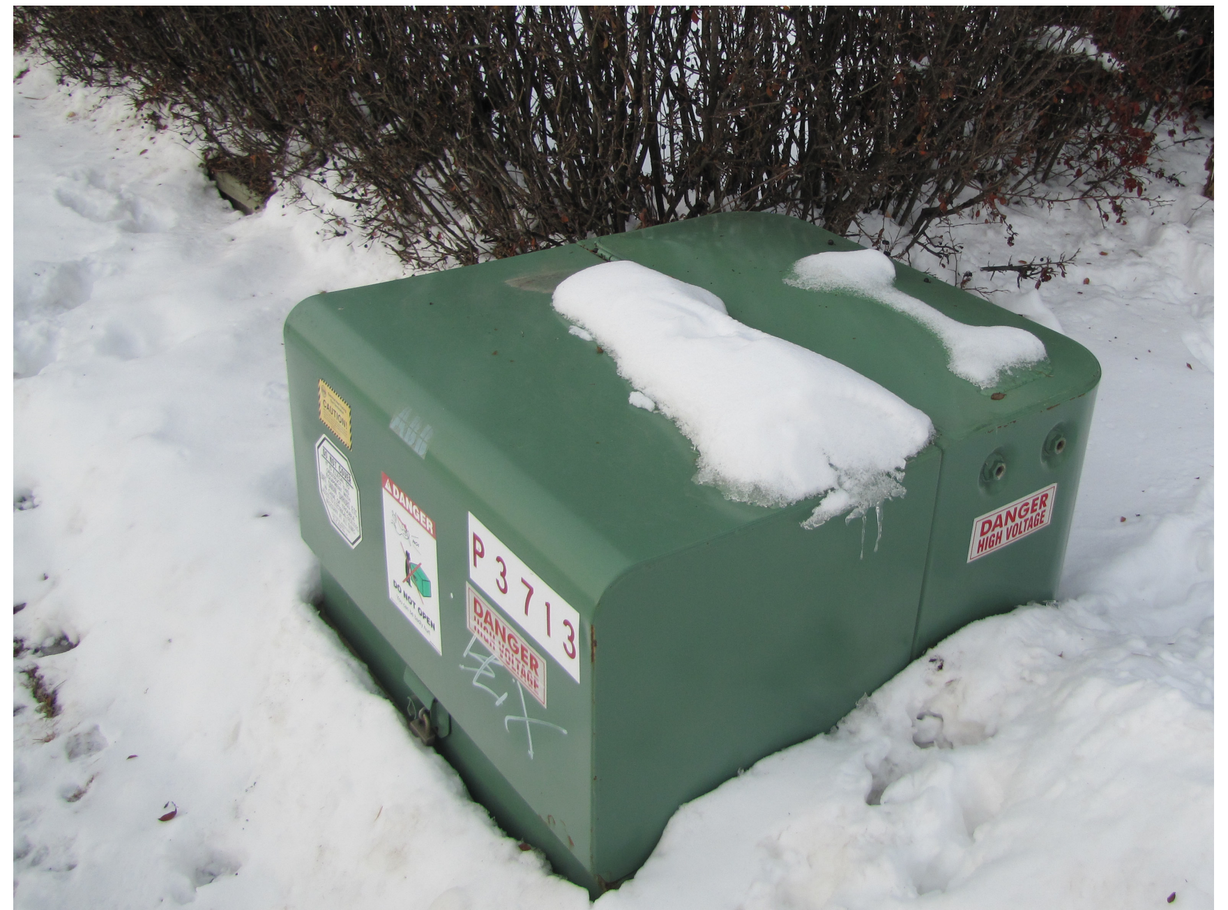
Phase Pad Mount Transformer
