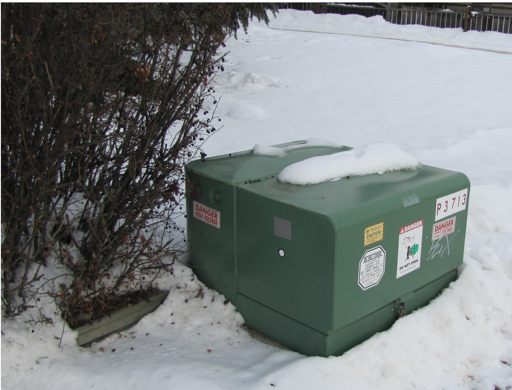
Phase Pad Mount Transformer
