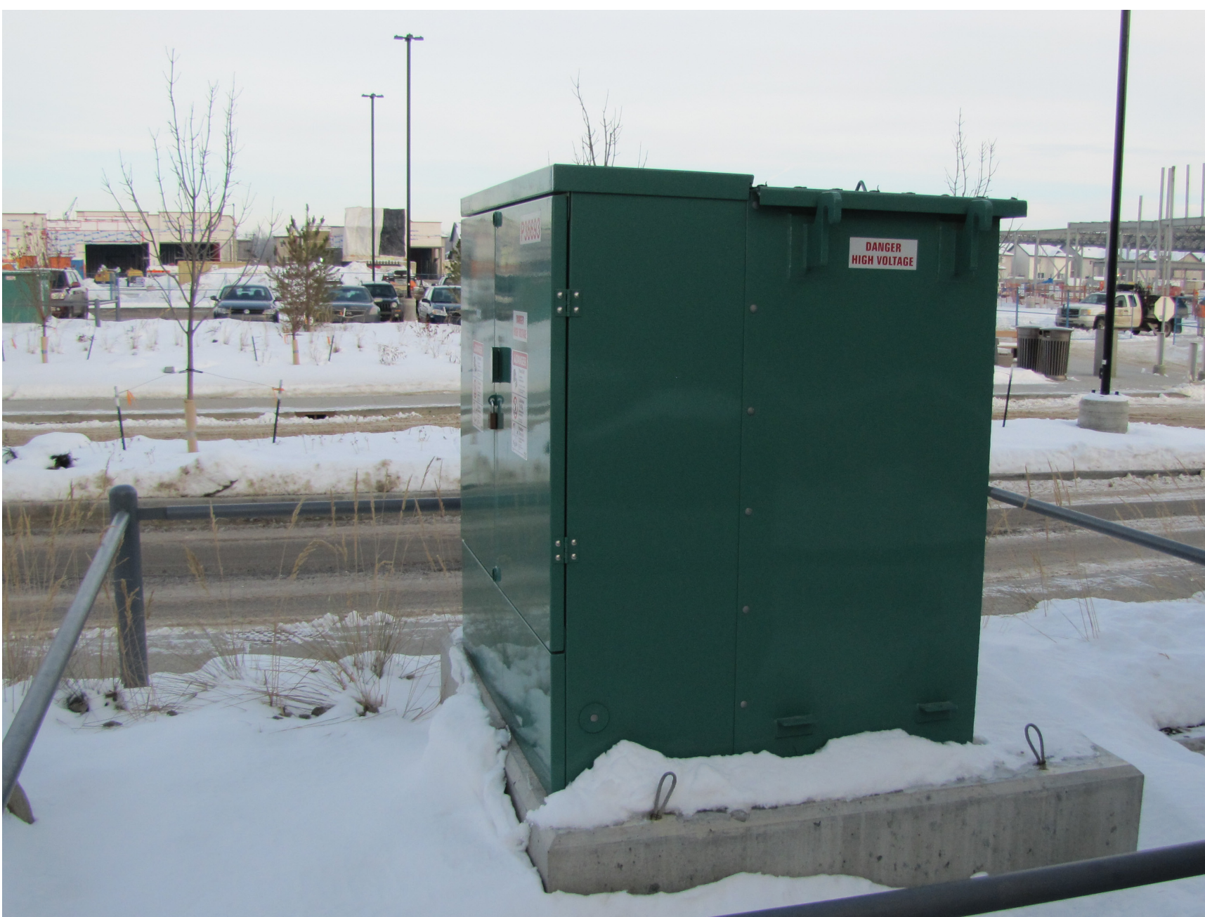
Phase Pad Mount Transformer
