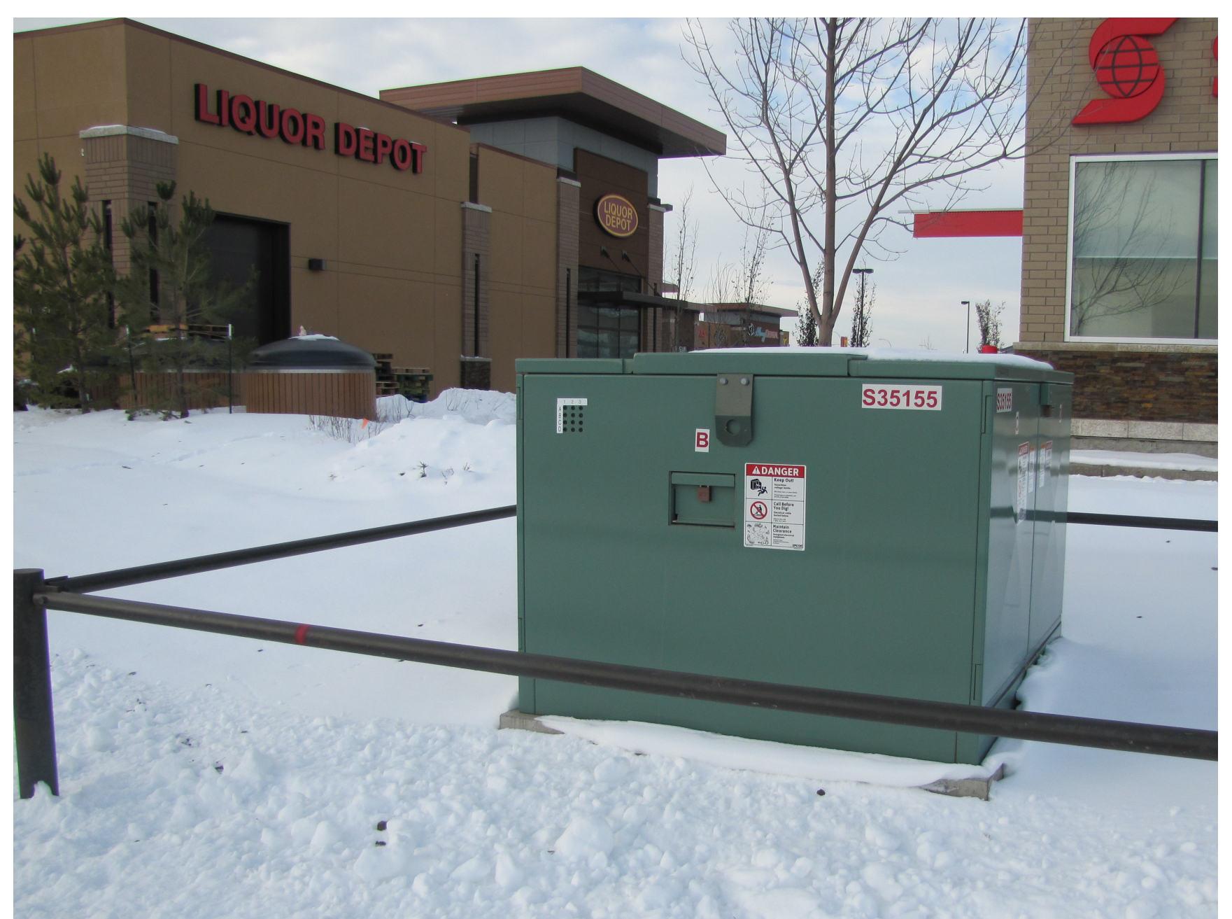
Switching Cubicle
