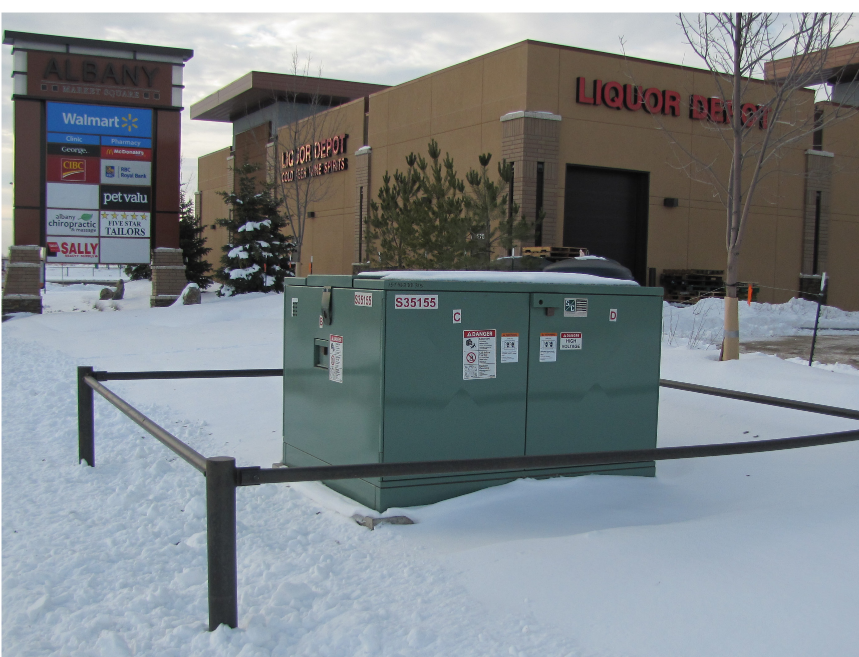
Switching Cubicle
