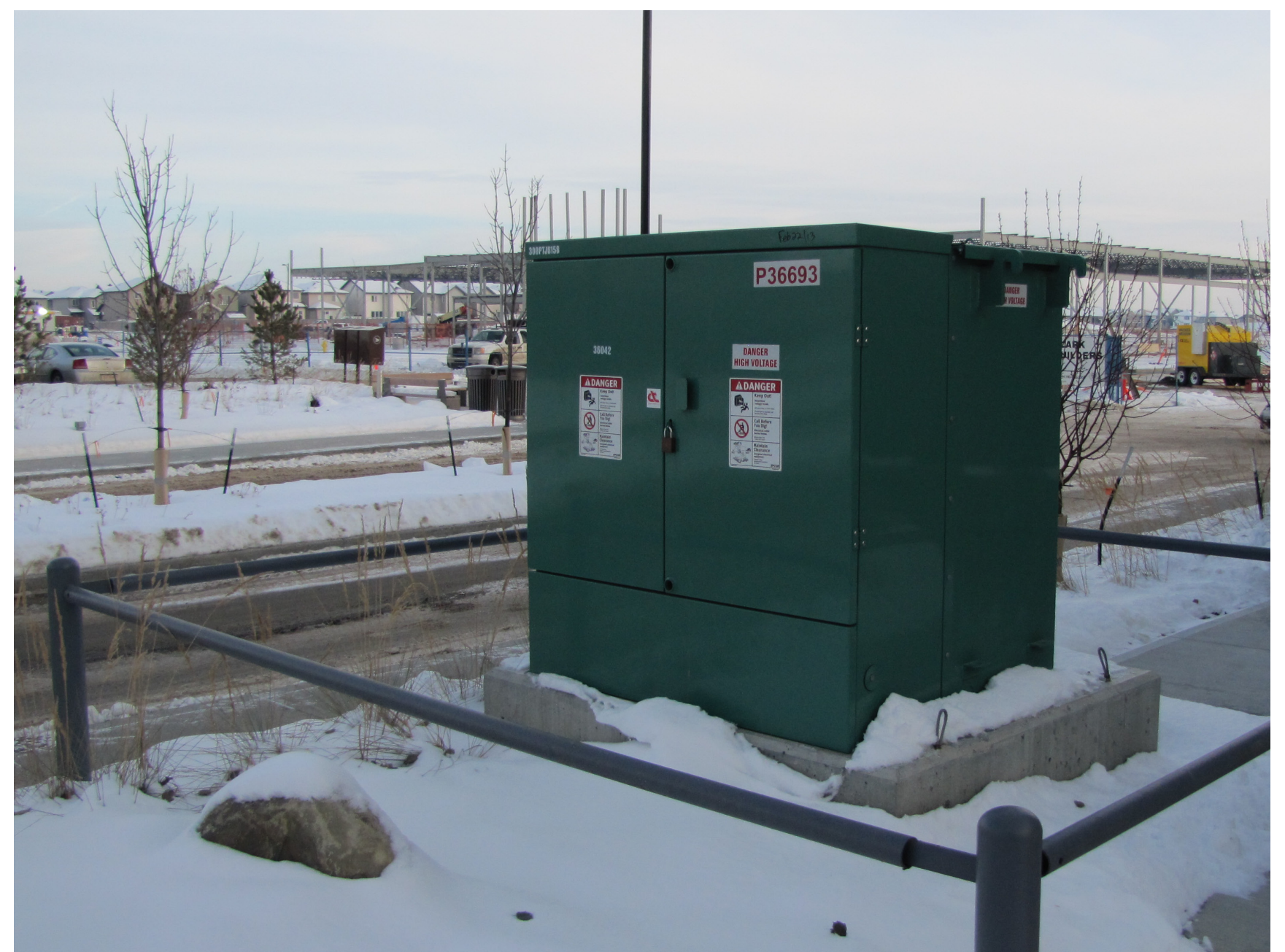
Phase Pad Mount Transformer
