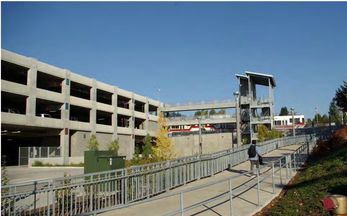
Figure 2.1: Park and Ride Site at Clackamas Town, Portland, OR, USA
