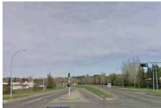
View A - Existing Condition
