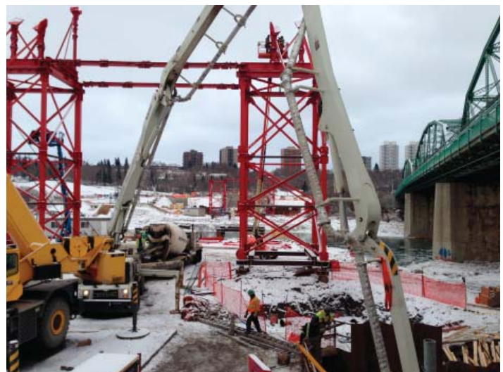
Crews assemble temporary lift towers
