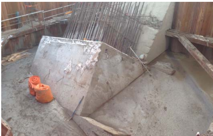
Backfilling the northwest cofferdam
