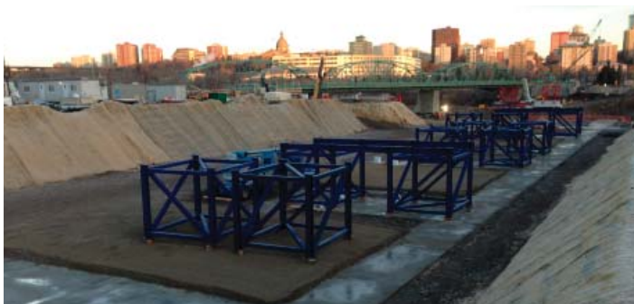
Tracks being set up in laydown area
