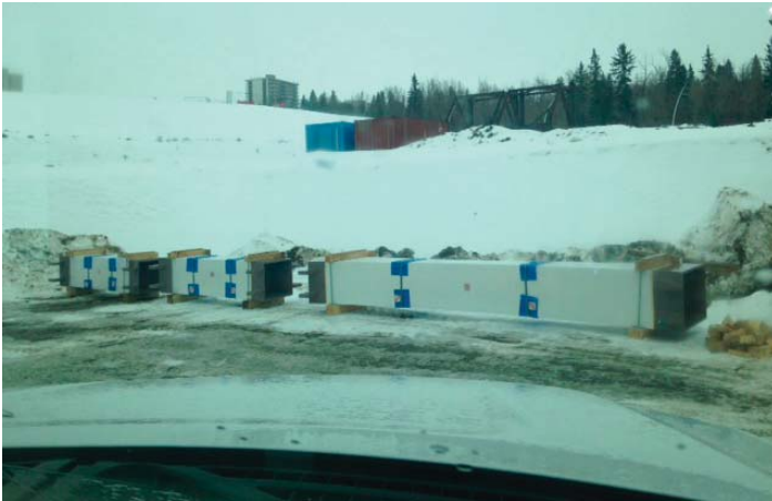
Arch struts arrive on site—January 2015
