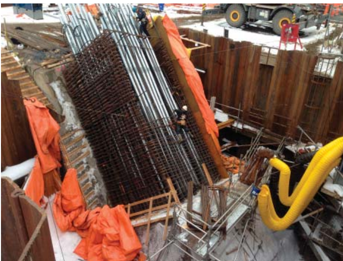
Workers placing rebar for the concrete bridge support legs
