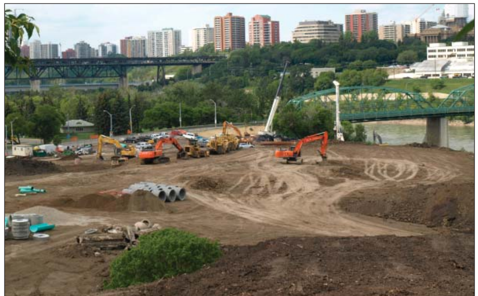
View of south side construction area from Queen Elizabeth Park
