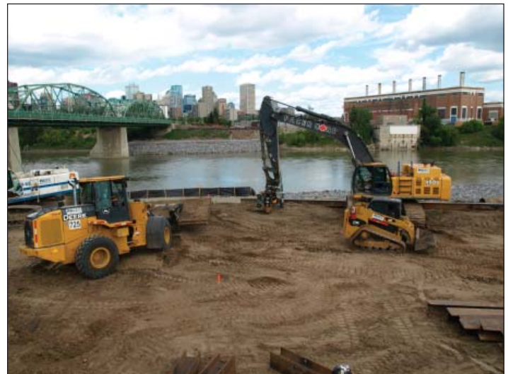
South side river bank construction
