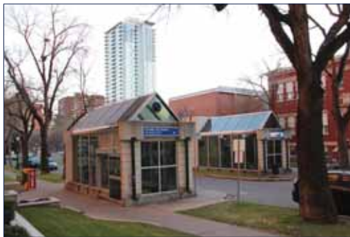
Pedestrian entrance at Grandin station
