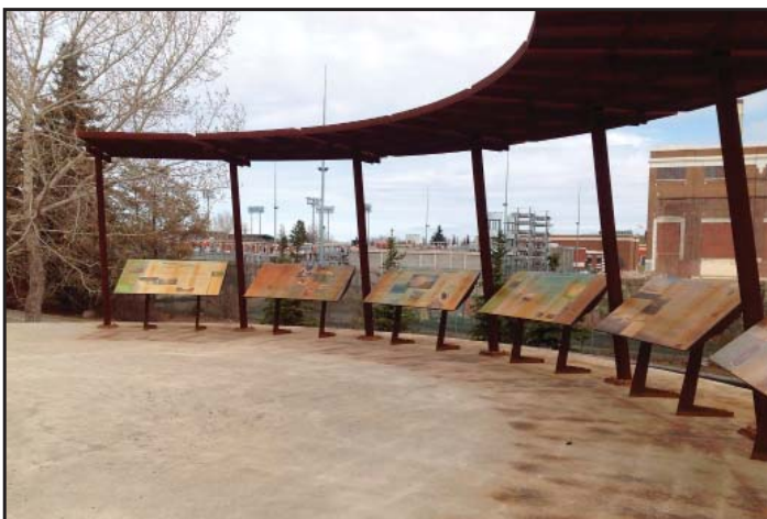
Interpretive Belvedere prior to relocation
