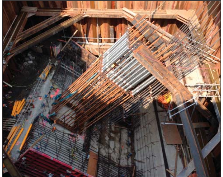
Anchor rods will support bridge arches
