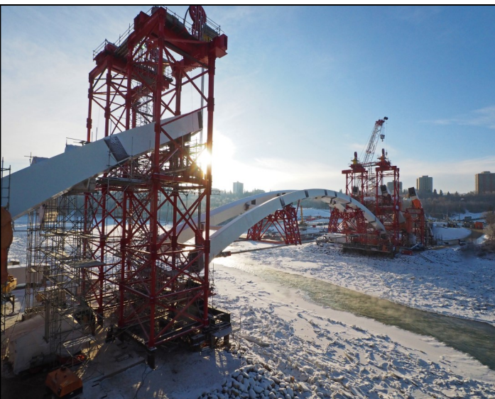
The arches being lifted into place
