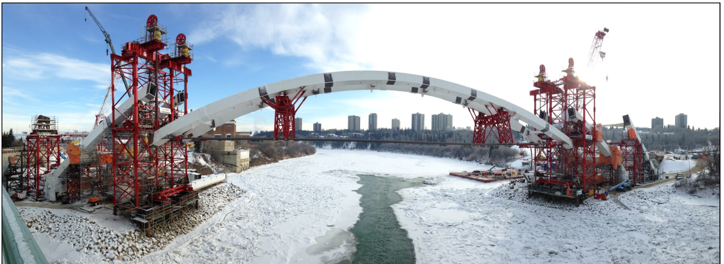
First arch lift completed
