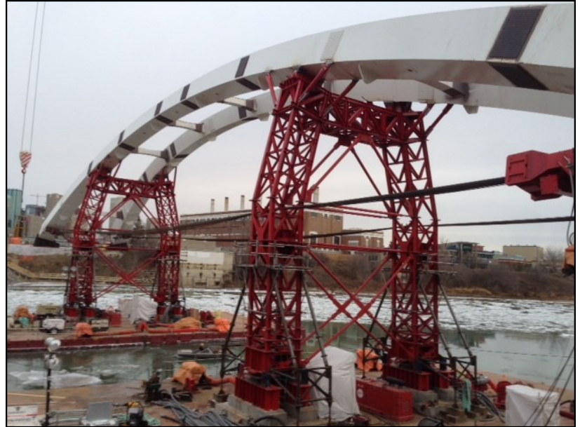
Central arch pieces are loaded onto the barges
