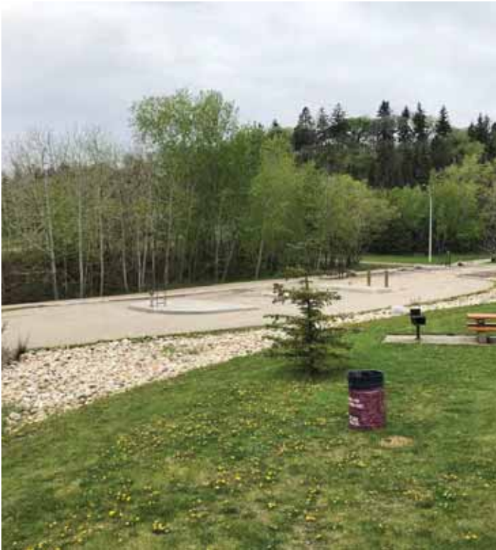
GROAT RAVINE TREATMENT FACILITY
