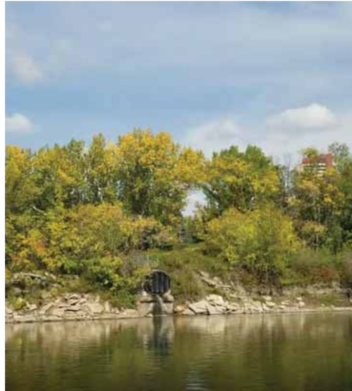
GROAT RAVINE STORMWATER OUTFALL
