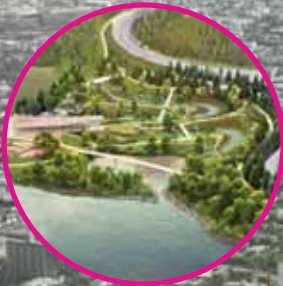
GROAT RAVINE DAYLIGHTING
