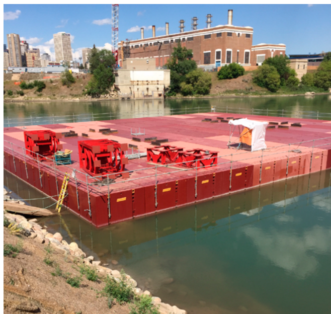
The assembled barge in south side laydown area
