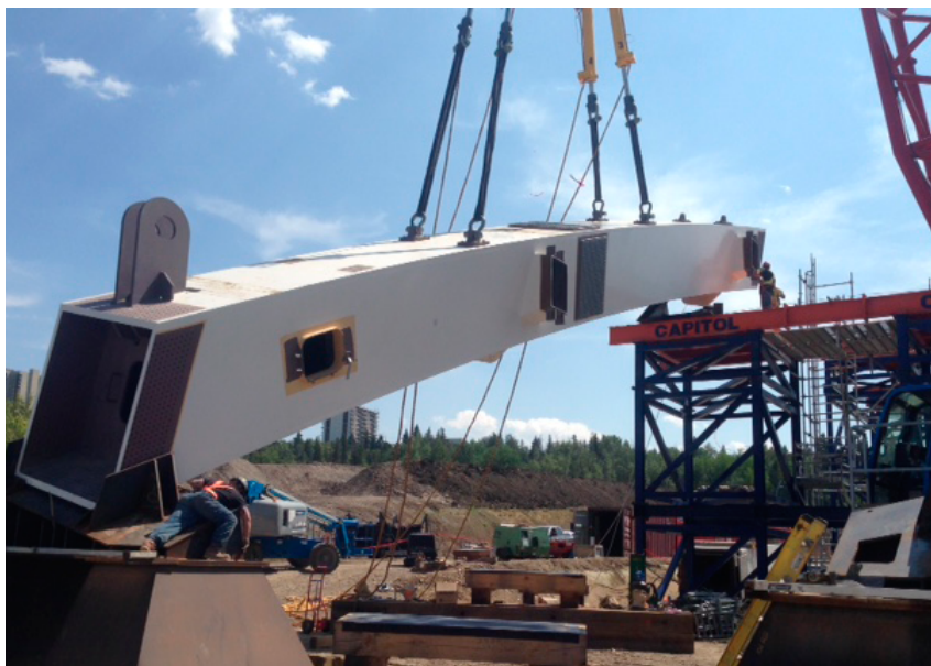
A piece of the central arch is moved during assembly
