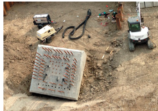
One of the backfilled cofferdams
