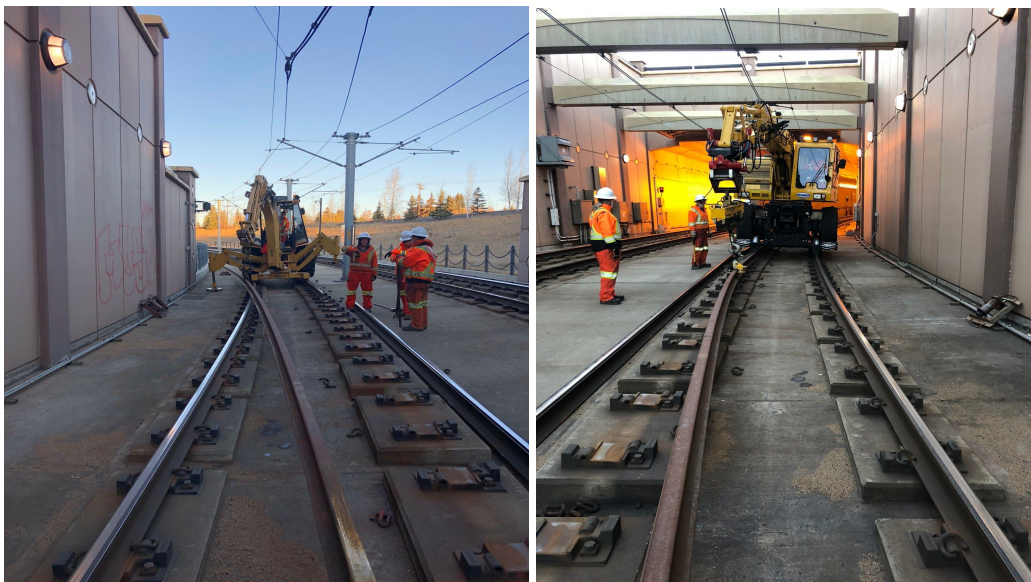
Pictures from the weekend of Oct 20-21 rail replacement work.
