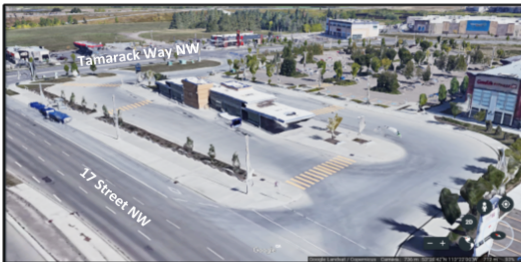
Figure 3.2-1 Meadows Transit Centre (Taken from Google Earth, 2018)
