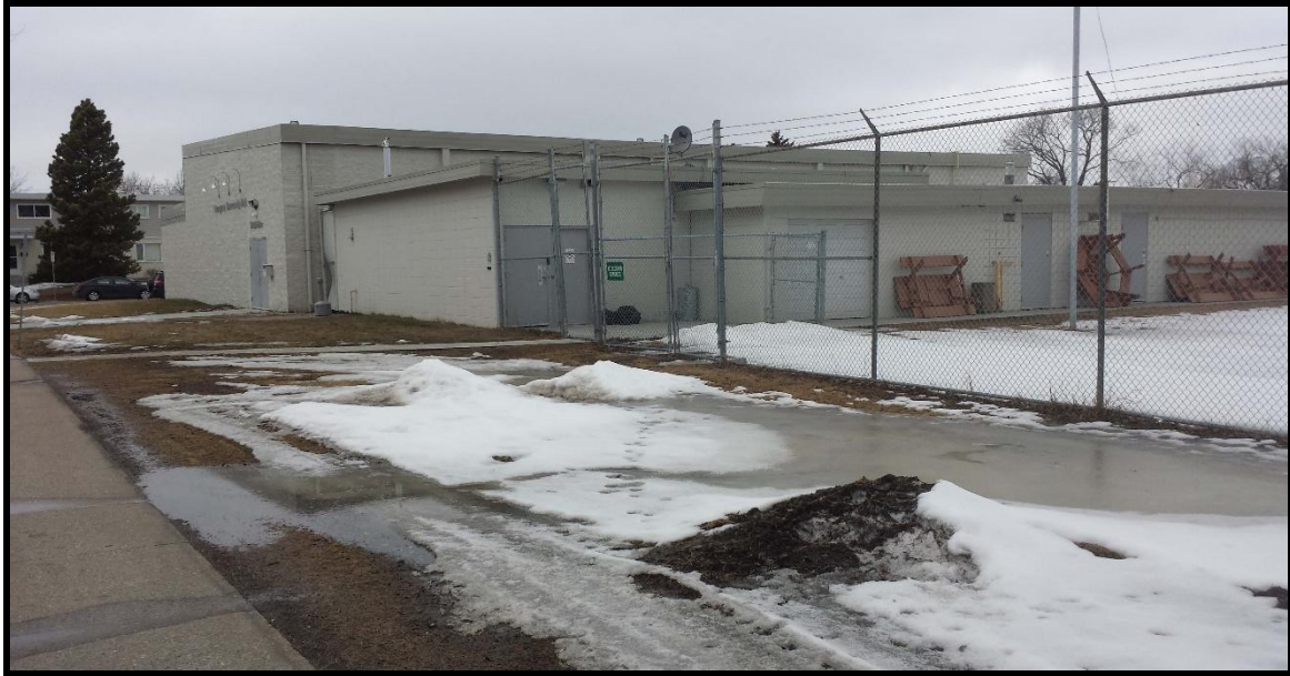
Figure 5.13 – Glengarry Community Hall fencing
