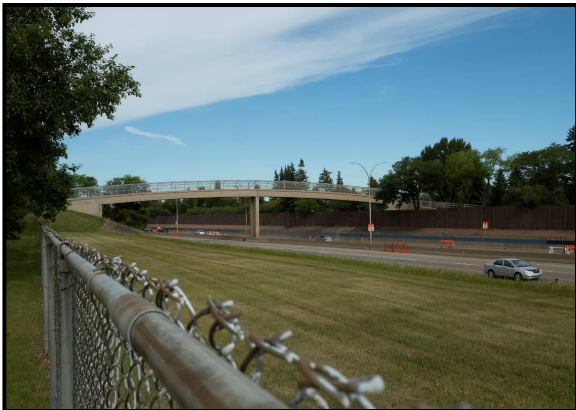
Figure 5.6: Whitemud Pedestrian Overpass
