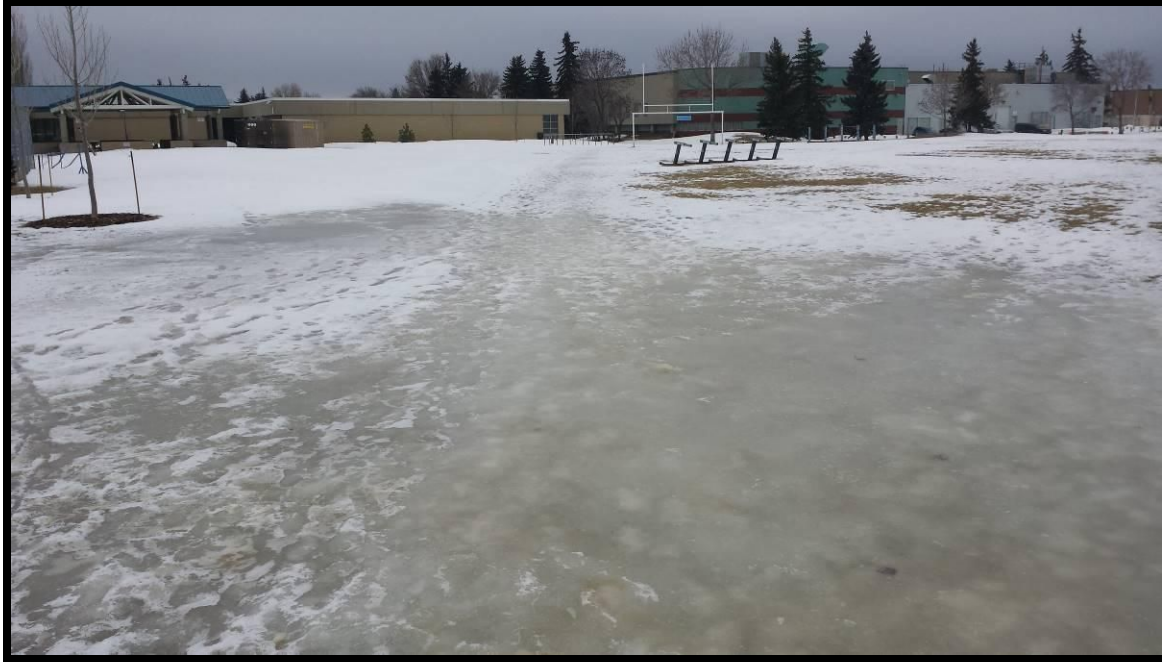
Figure 5.23: Field Drainage Issues
