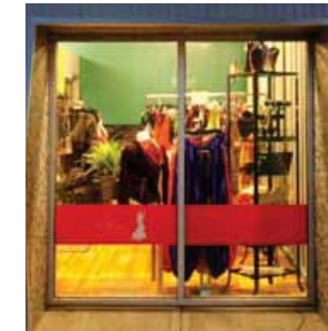
11805 - 94 Street Façade Improvement
