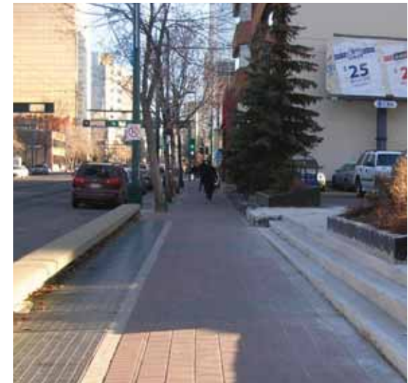
▲ The existing streetscape along Jasper Avenue is dated and deteriorated.
