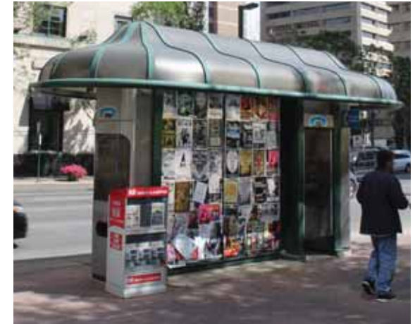
▲ Existing Utility Kiosk along Jasper Avenue
