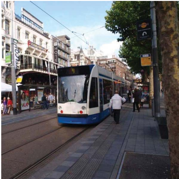
Figure 25: Low-Floor LRT - Amsterdam, Netherlands
