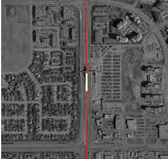
Figure 17: Infill Station Area
