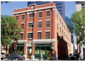
unusual combination of occupancies for the time. The structure is steel frame for all floors, which was also relatively unusual for the time since most Edmonton residential structure did not use steel framing past the first floor.
