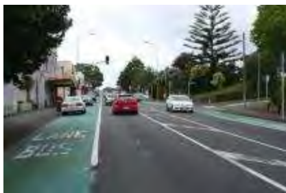
Bus service bus lanes open only in peak periods in Auckland, New Zealand
