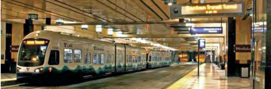
Figure 9 - Downtown Seattle Transit Tunnel
