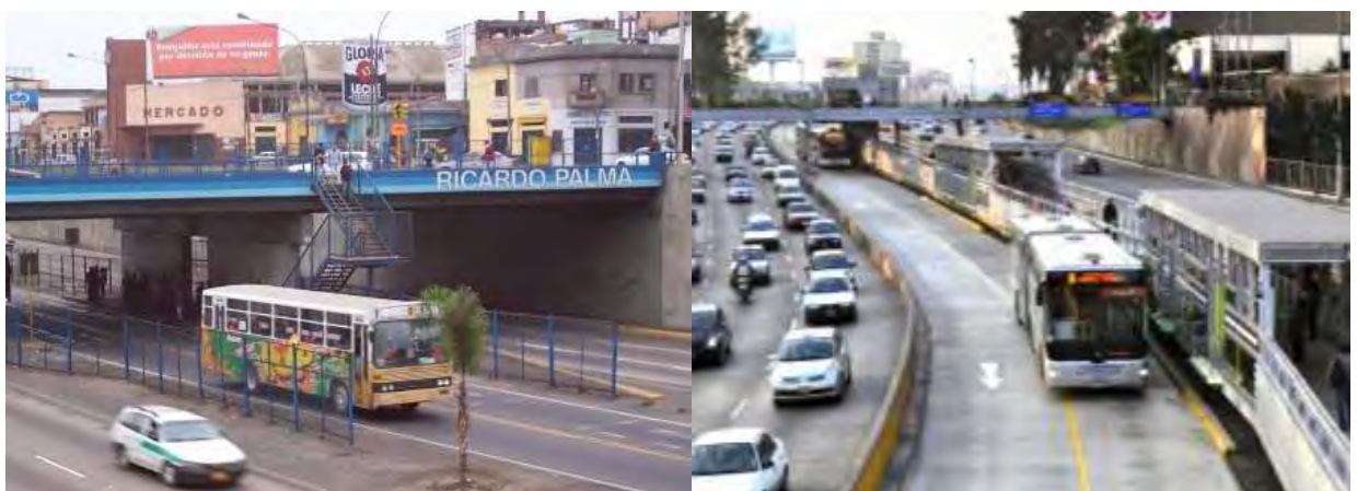
Figure 4 - El Metropolitano busway in the median in Lima, Peru
