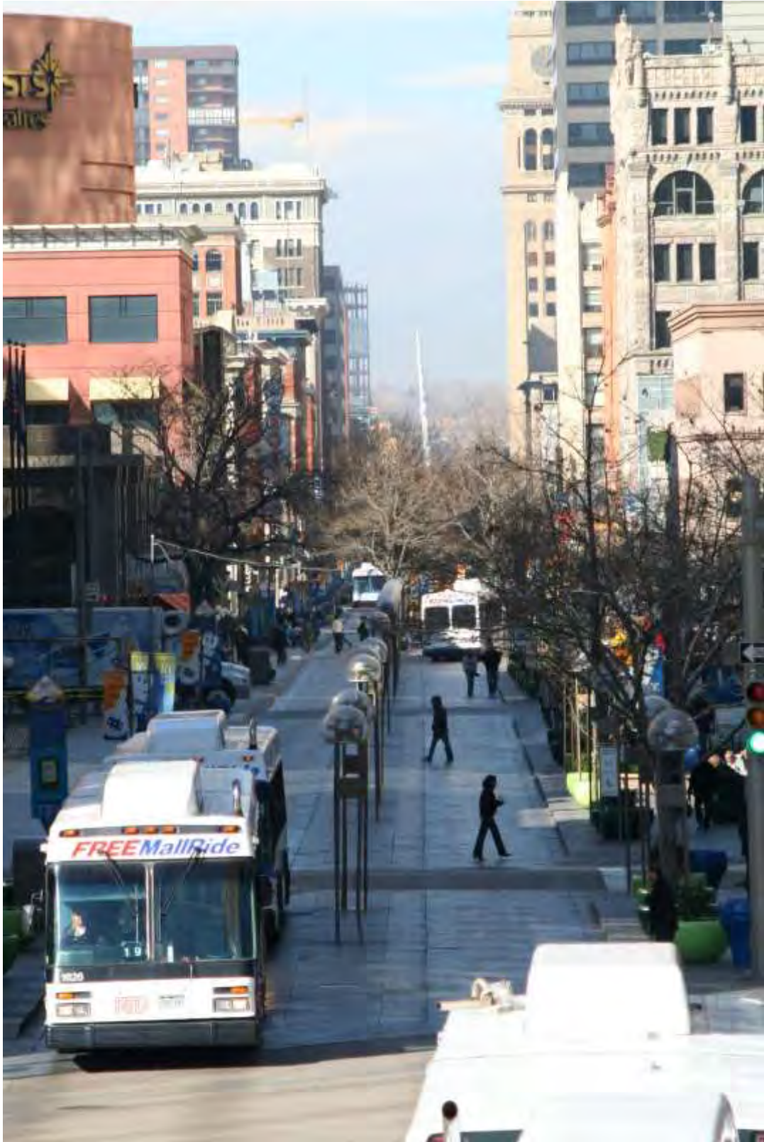
In 2014 there were at least 186 cities in the world with some type of bus priority system carrying nearly 32 million passengers per day. Bogotá's TransMilenio system (top and bottom left, front cover) stands out as one of the world's most recognisable Bus Rapid Transit (BRT) systems, however modest transit priority corridors such as Denver's 16 th Street Mall (above), with specialty vehicles, frequent service, and dedicated bus lanes, can also have substantial benefits.
