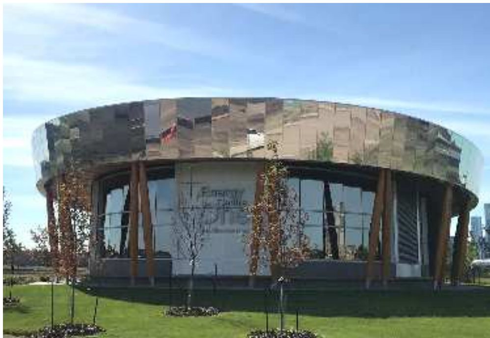
Energy Centre One harnesses earth's geothermal renewable energy for use in the community's District Energy Sharing System.
